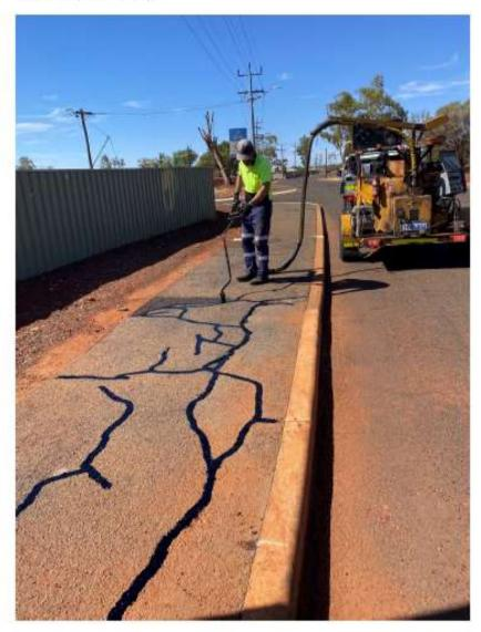
Photo attached of sealant being poured on Phoenix Street footpath near Duketon St intersection.
