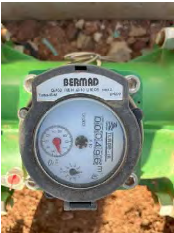
Figure 1.8 Standpipe Discharge Flowmeter Details-1
