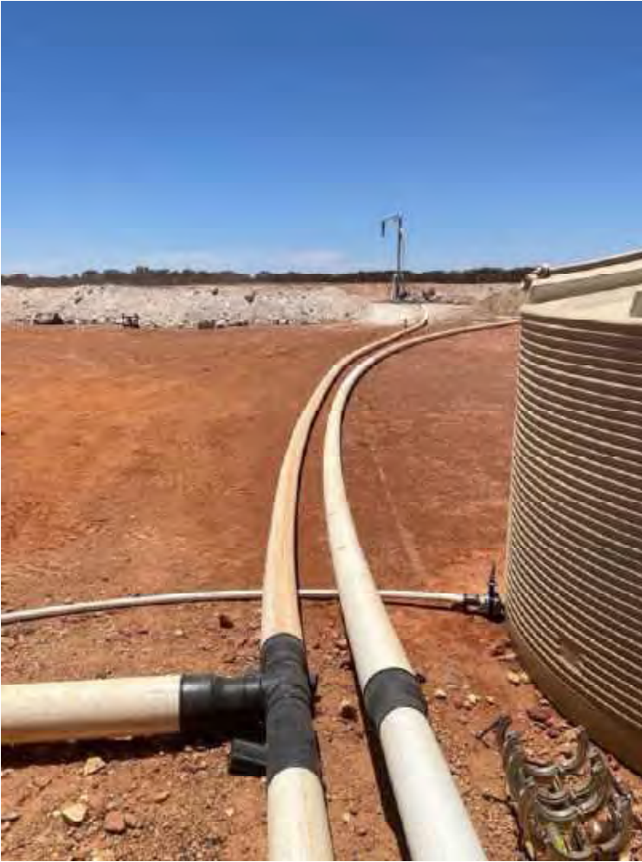
Figure 3: Dewatering from Turkey Nest - Standpipes Line (left) and Mesa Discharge Line (right)
