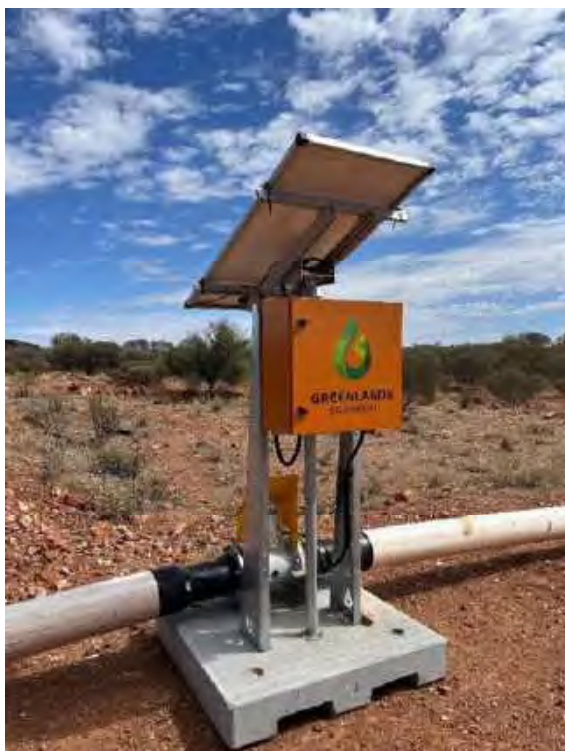
Figure 1.3 Mesa Telemetry Panel
