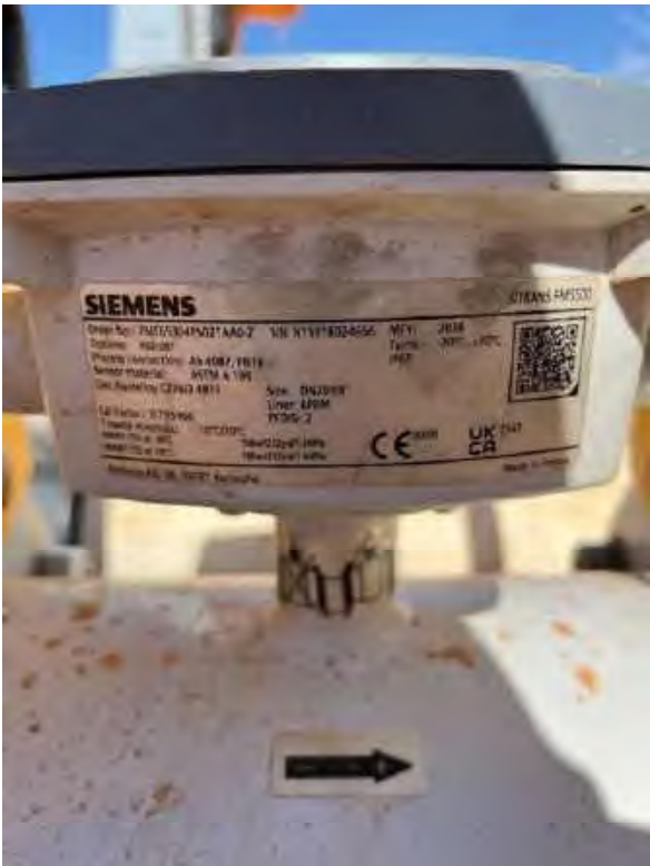
Figure 1.7 South Pit Abstraction Flowmeter Details
