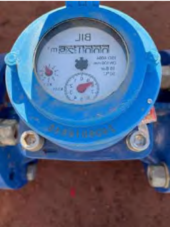
Figure 1.8 Standpipe Discharge Flowmeter Details-1
