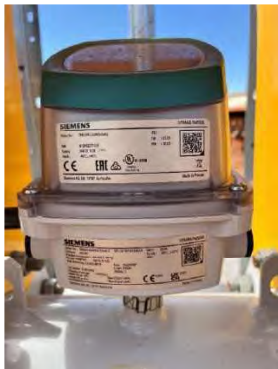
Figure 1.4 Mesa Discharge Flowmeter Details
