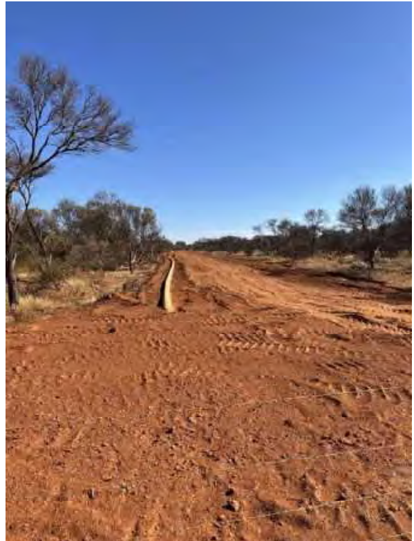
Figure 1.10 Mesa Transfer line in V-drain
