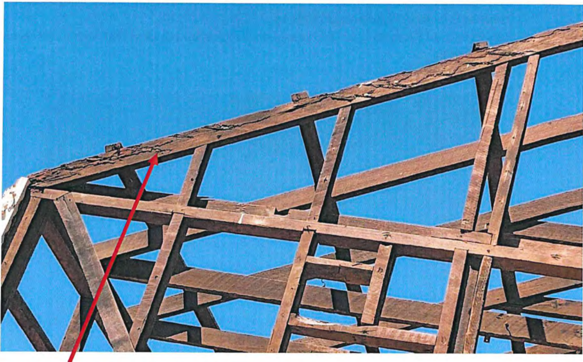
Termite damage to several rafters visible
