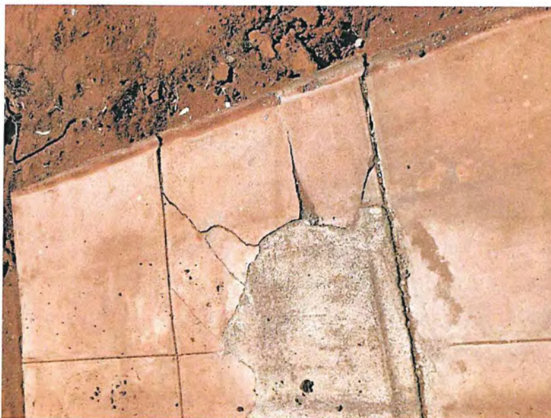
Rear slab on ground, badly cracked
