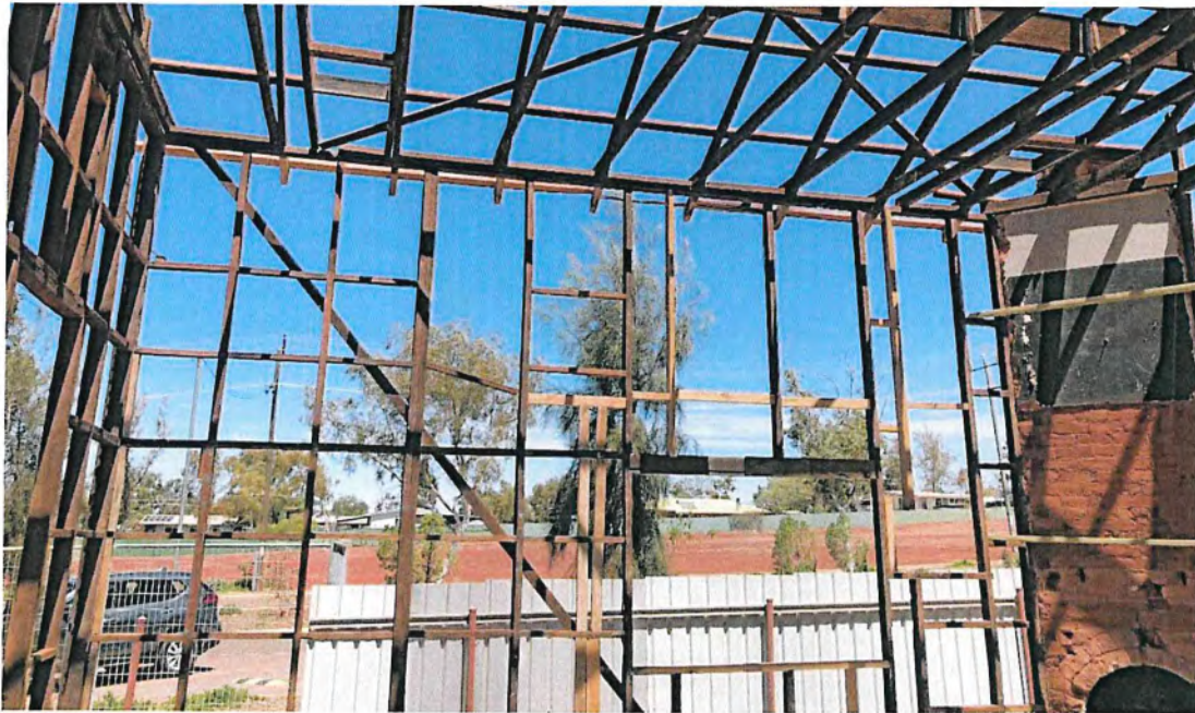
The timber framing has been modified during its lifetime
