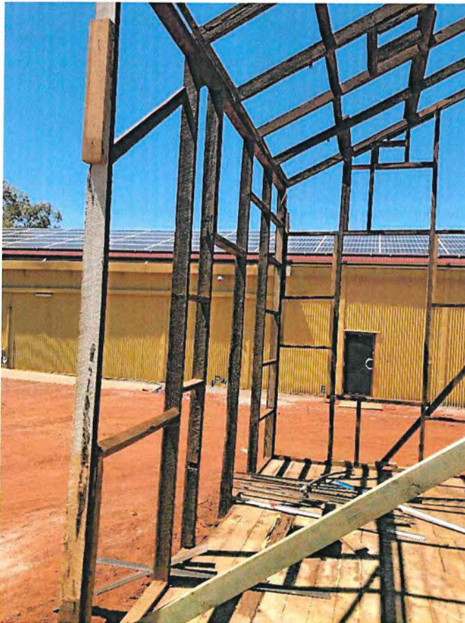
Numerous timber elements with termite attack visible
