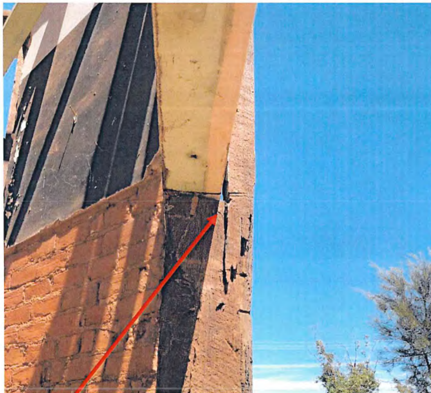
Notched and split timber stud
