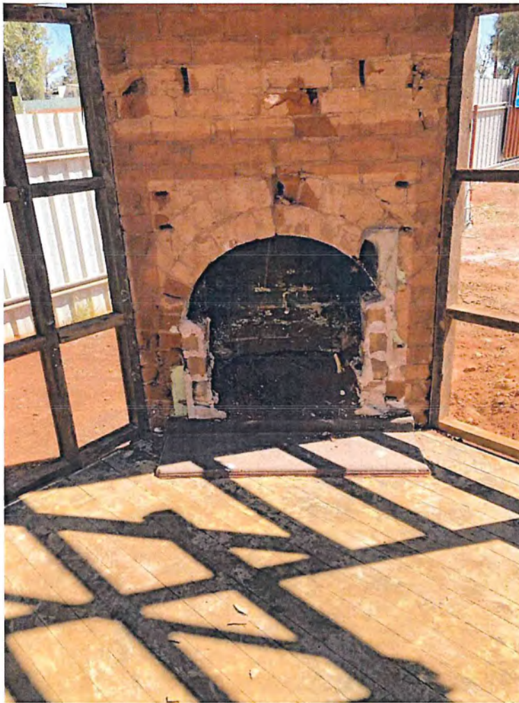
The chimney is no longer capable of providing horizontal support to the building frame
