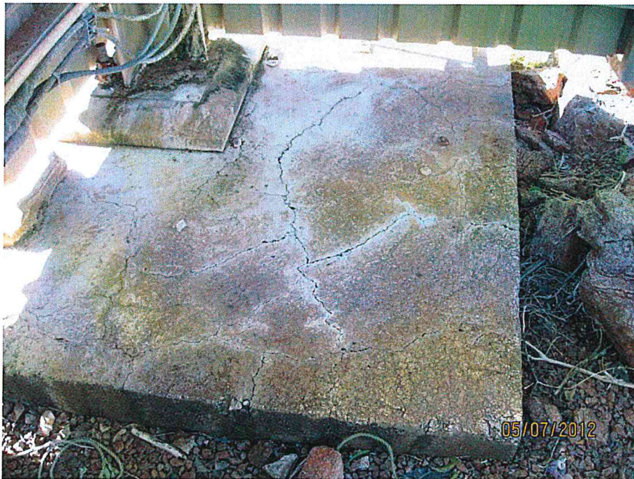
Figure 8 – Footing cracks.
