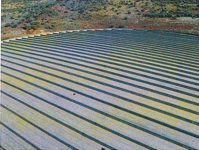
Figure 23 - Tank roof sheeting.
