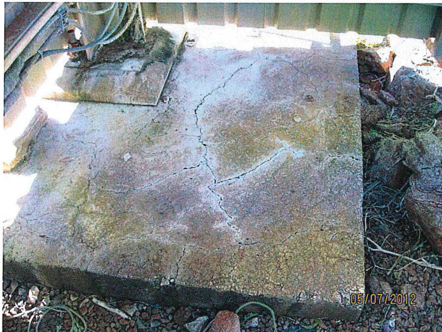
Figure 8 – Footing cracks.
