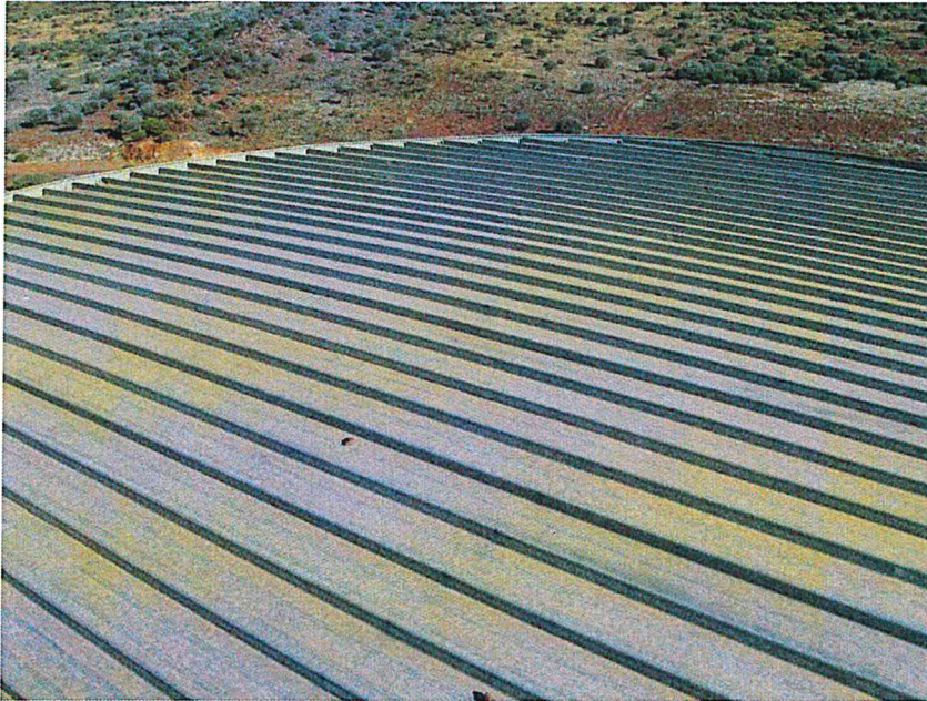
Figure 23 - Tank roof sheeting.
